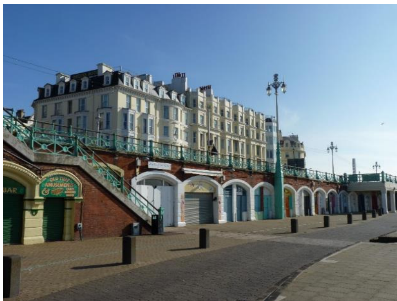
Brick arches supporting King's Road
