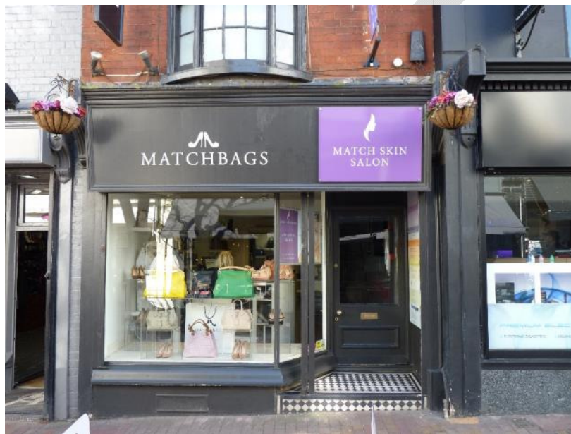
Duke Street: traditional shopfront details obscured by an over-deep fascia
