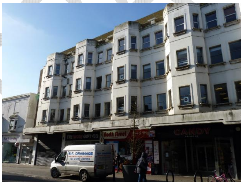
Nos.21-25 North Street
